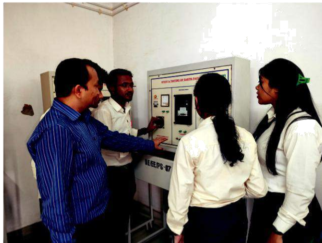
Power System Lab
